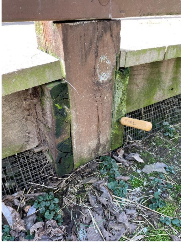
Photo 7 – Rotted 2x10 side members of built-up wood girder w/embedded ice pick
